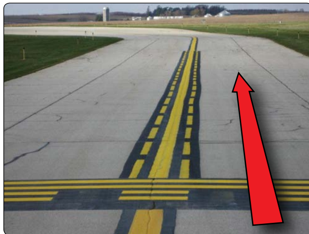
Figure 1-24. Runway holding position markings as seen when exiting the runway. When exiting the runway, no ATC clearance is required to cross.
