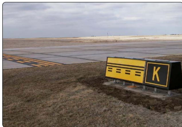
Figure 1-27. Runway safety area boundary sign and marking located on Taxiway Kilo.
