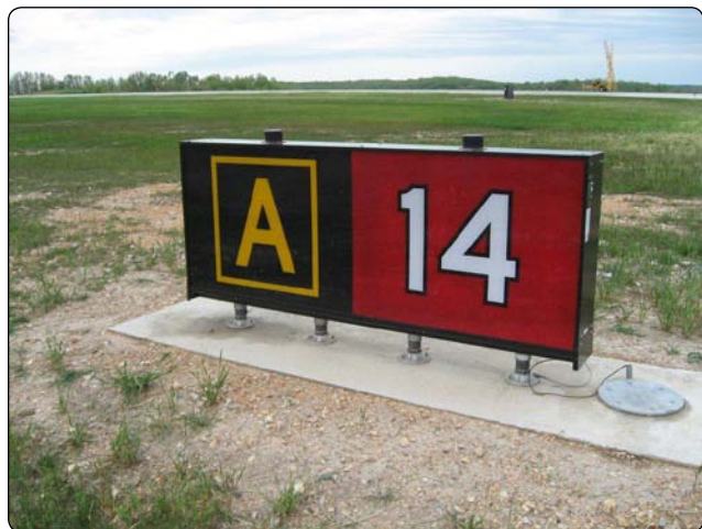
Figure 1-19. Runway holding position sign at takeoff end of Runway 14 with colocated Taxiway Alpha location sign.
