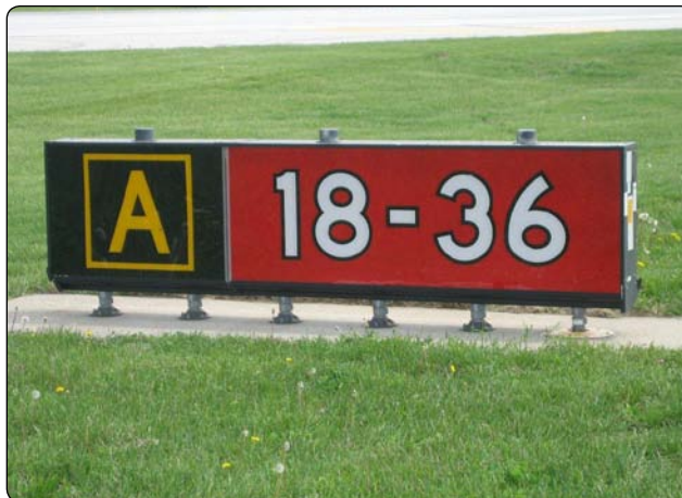
Figure 1-20. Runway holding position sign at a location other than the takeoff end of Runway 18-36 with colocated Taxiway Alpha location sign.
