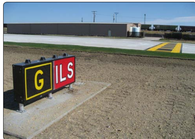
Figure 1-36. Instrument landing system (ILS) holding position sign and marking on Taxiway Golf.
