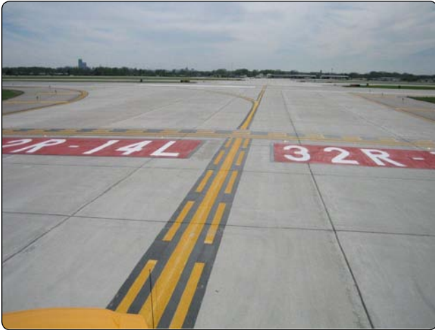
Figure 1-22. Surface painted runway holding position signs for Runway 32R-14L along with the enhanced taxiway centerline marking.
