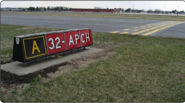
Figure 1-37. Runway 32 approach area sign and marking on Taxiway Alpha.
