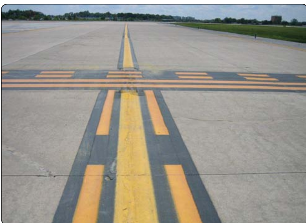
Figure 1-23. Surface painted holding position marking along with enhanced taxiway centerline.
