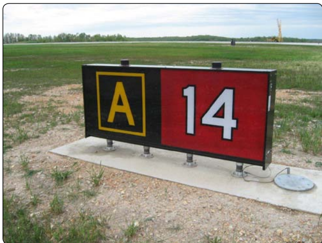
Figure 1-19. Runway holding position sign at takeoff end of Runway 14 with collocated Taxiway Alpha location sign.
