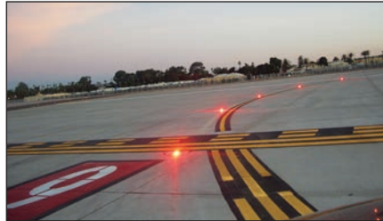
Enhanced taxiway centerlines are designed to reduce pilot deviations.
