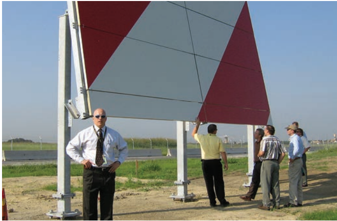
FAA Engineering Psychologist Mark Reisweber stands in front of an End-Around Taxiway masking screen at DFW.
