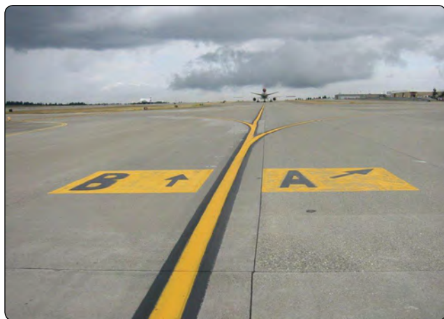
Figure 14-19. Surface painted taxiway direction signs.
