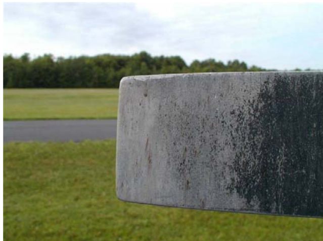
FIGURE 1-7. Erosion on a Metal Blade
