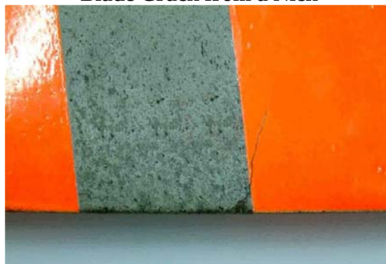
FIGURE 1-9. Blade Crack from a Nick
